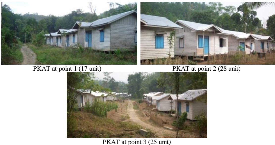
Figure 11 resettlement program at Kamawakan village Source: documentation, 2011.
